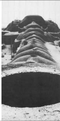
Kashan, roofscape of the bazaar
