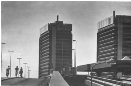
Jaap Rozema, 1979, Prins Bernhardviaduct
