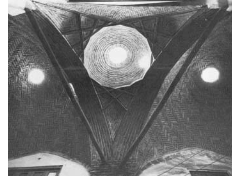
Isfahan brick ceiling of bazaar route
